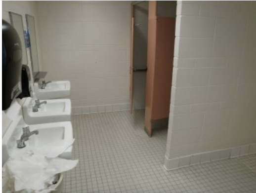
Figure 7, renovated toilet room
