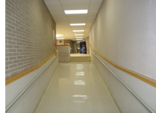
Figure 9, stair from east side entry to lecture hall.
