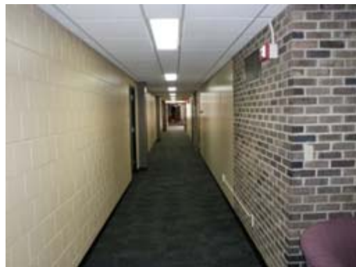
Figure 11, corridor in classroom wing.
