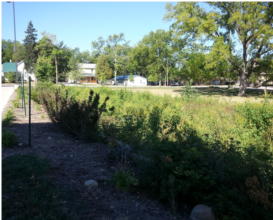
FIGURE 5 - LOT 2 BIORETENTION BASIN
