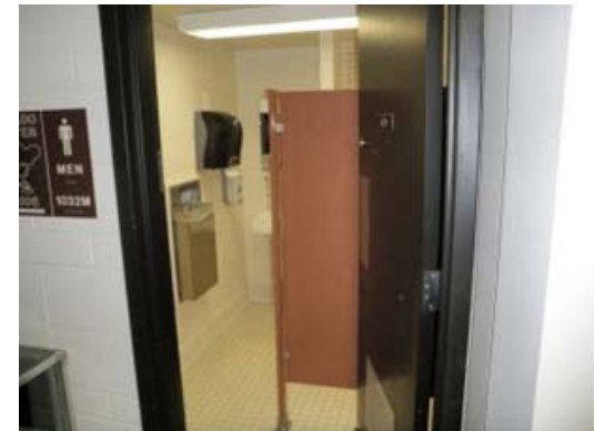
Figure 6, renovated toilet room
