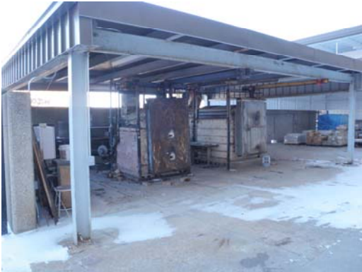
Figure 16, exterior kiln area
