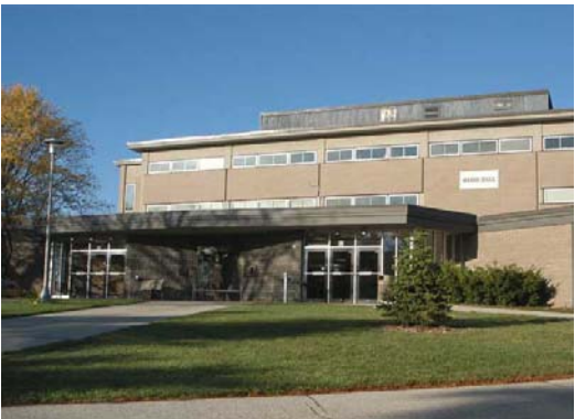
Figure 19, east entry of the building.
