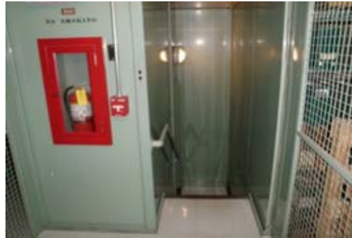
Figure 8, access stair in 1952 bldg high density storage.
