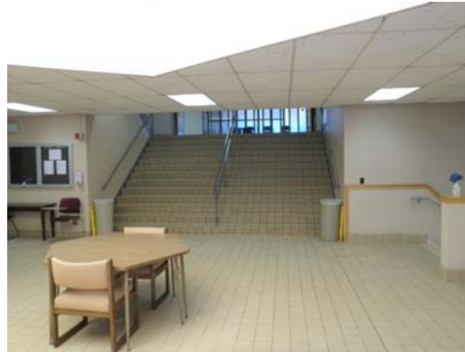
Figure 14, stairs from east main entry to first floor.
