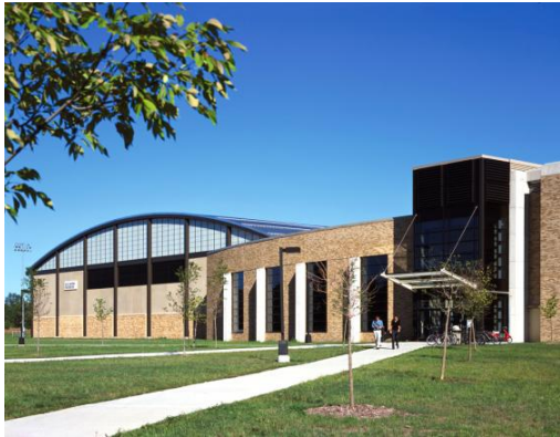
Figure 21, Kachel Fieldhouse, south building entry
