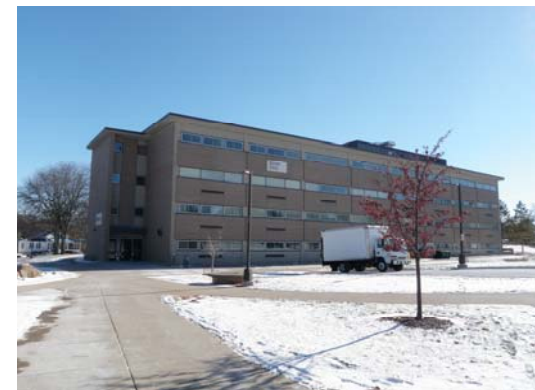
Figure 18, exterior view of the west side of the building.
