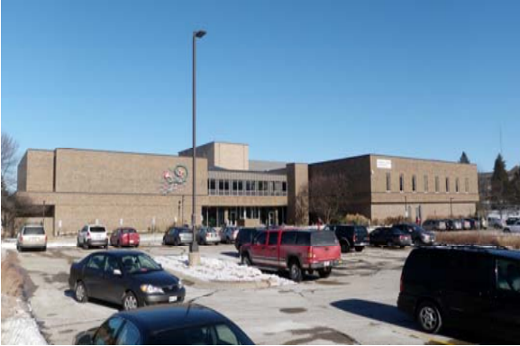
Figure 14, main entry on south side of building
