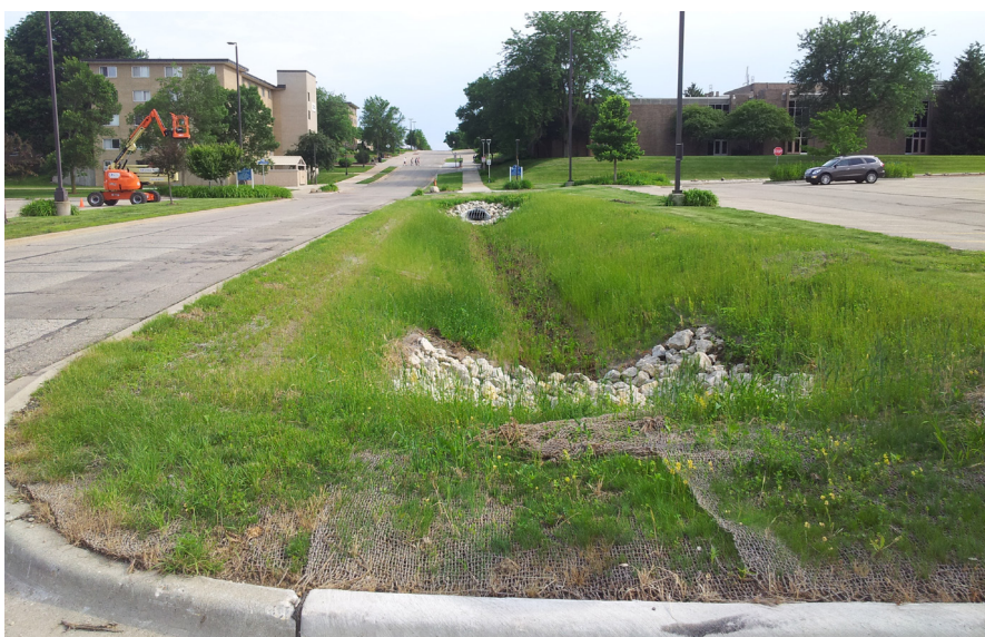
FIGURE 1 - FLOOD RELIEF BIOSWALE - PRAIRIE ST.
