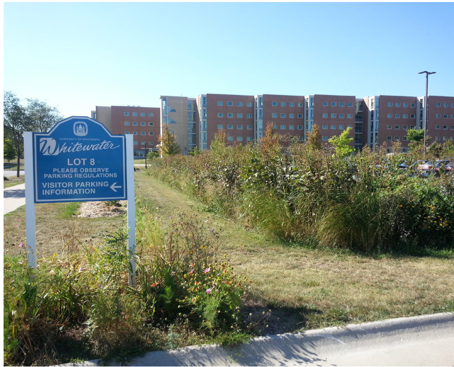
FIGURE 4 - LOT 8 BIORETENTION BASIN
