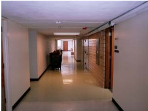
Figure 1, ground floor corridor between 1952 bldg and 1964 bldg.
