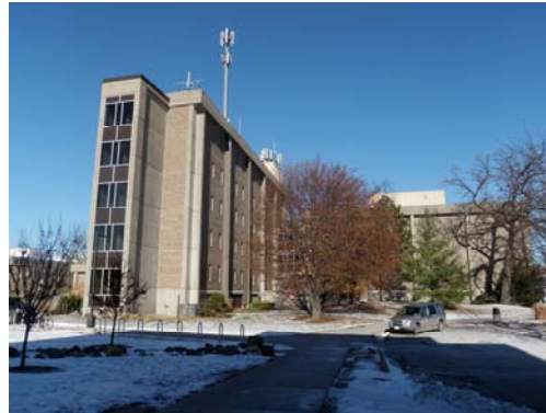
Figure 14, exterior view from southeast
