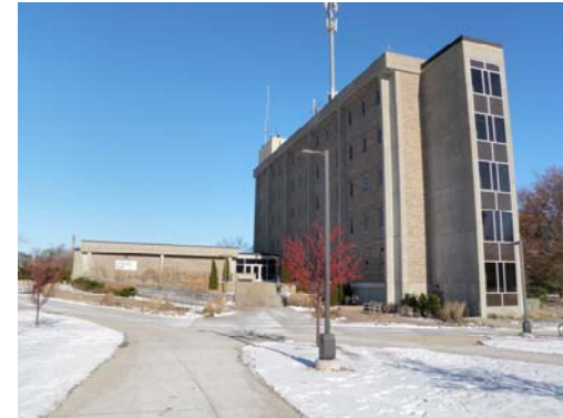
Figure 14, exterior view from southwest
