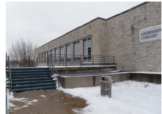
Figure 24, north face of 1952 building
