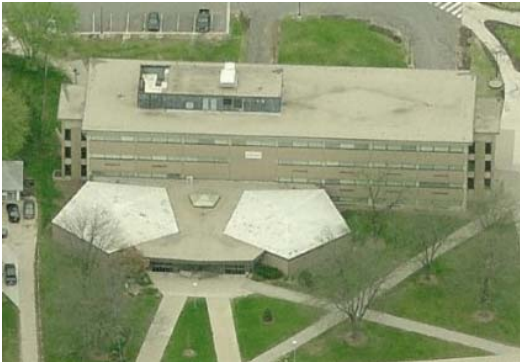
Figure 19, birdseye view of the east side of the building.
