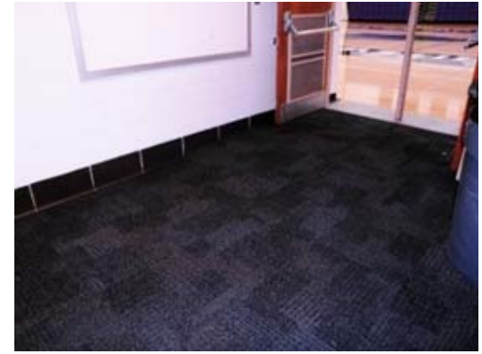
Figure 3, flooring at gym entry.
