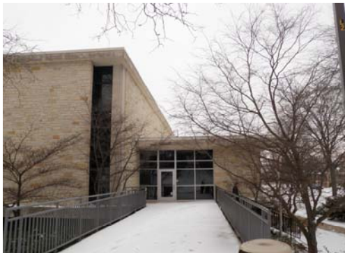
Figure 22, southwest corner of 1962 building
