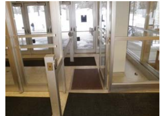
Figure 12, 1 st floor entry at link btwn 1951 and 1962 bldg.
