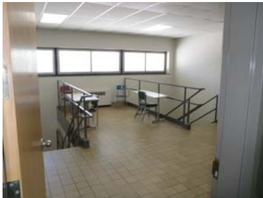
Figure 16, top landing of central stair.
