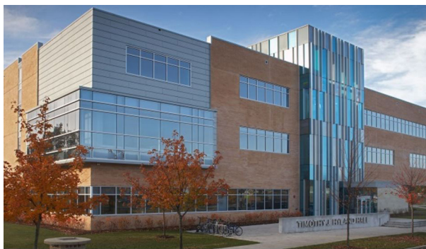
FIGURE 201: METAL PANEL AND MASONRY IN ACADEMIC PROJECTS
