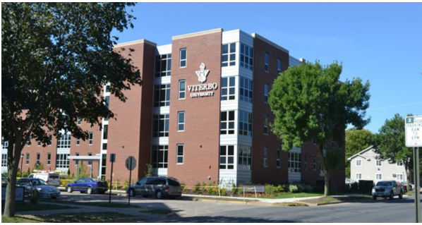
FIGURE 198: METAL PANEL AND MASONRY IN RESIDENTIAL PROJECTS
