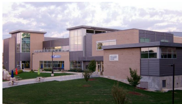
FIGURE 197: MIX OF METAL PANEL AND MASONRY IN NEW UNIVERSITY PROJECTS, CONNOR UNIVERSITY CENTER
