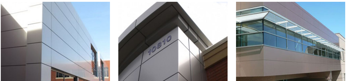
FIGURE 139, 140, 141: CLEAR ANODIZED METAL PANEL, METAL PANEL PLATINUM/ SILVER, MEDIUM CHAMPAGNE (LEFT TO RIGHT)
