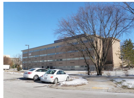
FIGURE 195 EXISTING MATERIALS, HEIDE HALL
