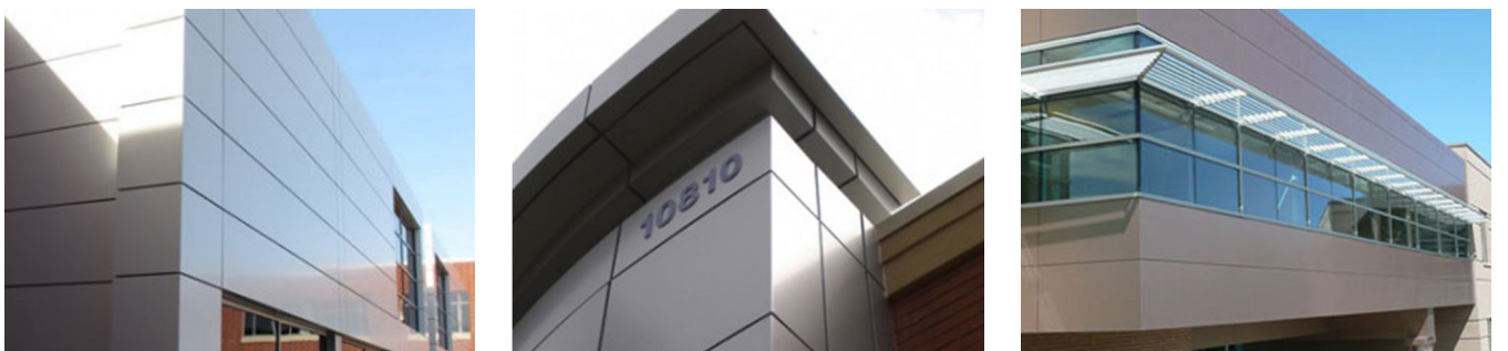
FIGURE 109, 110, 111: CLEAR ANODIZED METAL PANEL, METAL PANEL PLATINUM/ SILVER, MEDIUM CHAMPAGNE (LEFT TO RIGHT)
