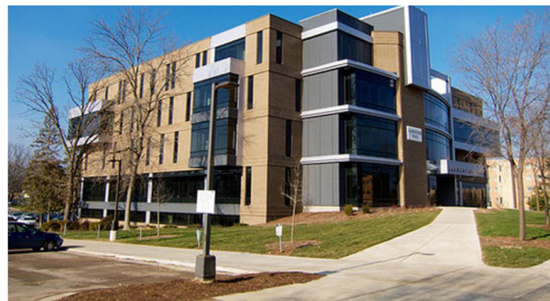
FIGURE 196: METAL PANEL USE IN RENOVATION PROJECTS, LAURENTIDE HALL
