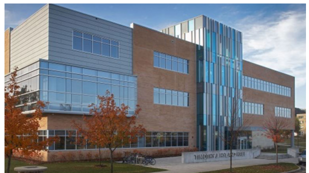
FIGURE 185: ROOF FORM ON ACADEMIC BUILDINGS
