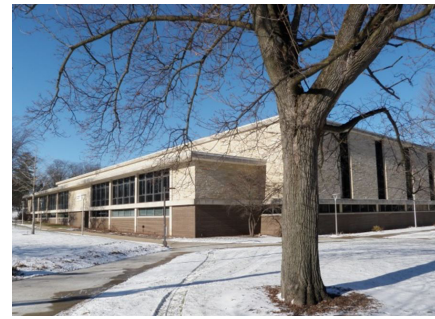
FIGURE 194: EXISTING MATERIALS, ANDERSEN LIBRARY
