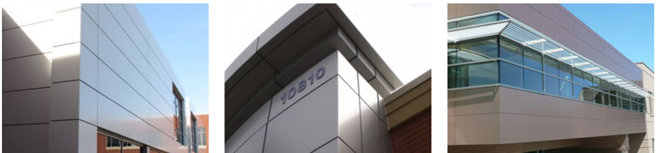
FIGURE 123, 124, 125: CLEAR ANODIZED METAL PANEL, METAL PANEL PLATINUM/ SILVER, MEDIUM CHAMPAGNE (LEFT TO RIGHT)
