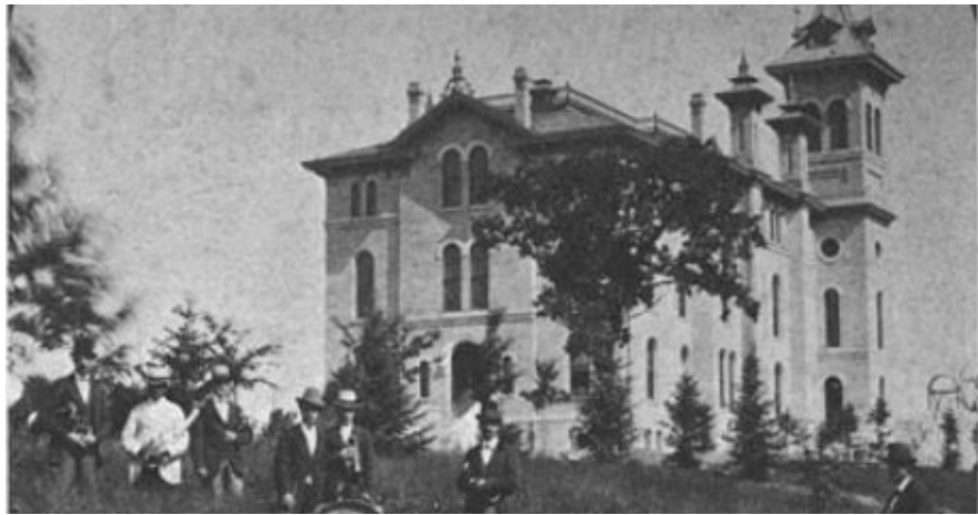
FIGURE 16: OLD MAIN HALL WITH NORTH WING ADDITION CIRCA 1876
